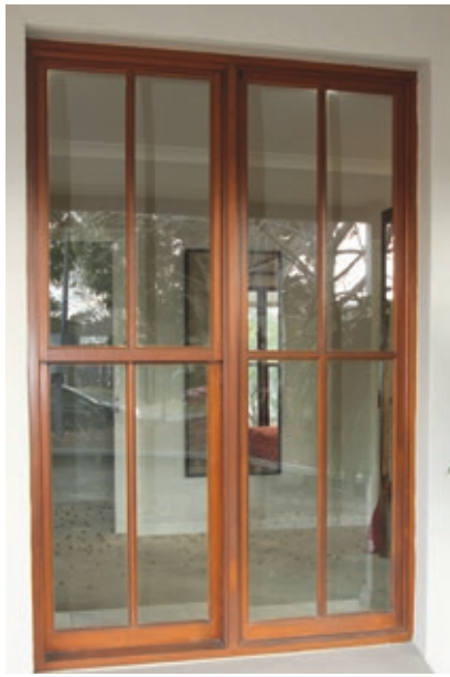
Western Red Cedar window upgrade
